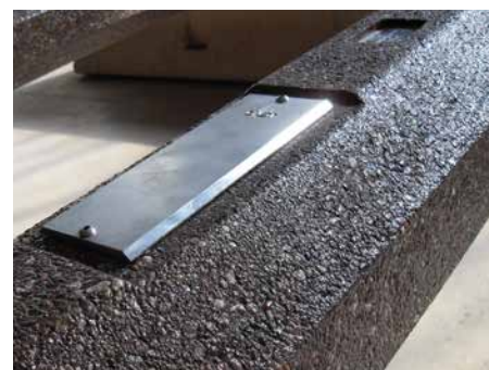
Detail eines Schleuderbeton-Strommasts Detail of an Electrical Spun Pole
