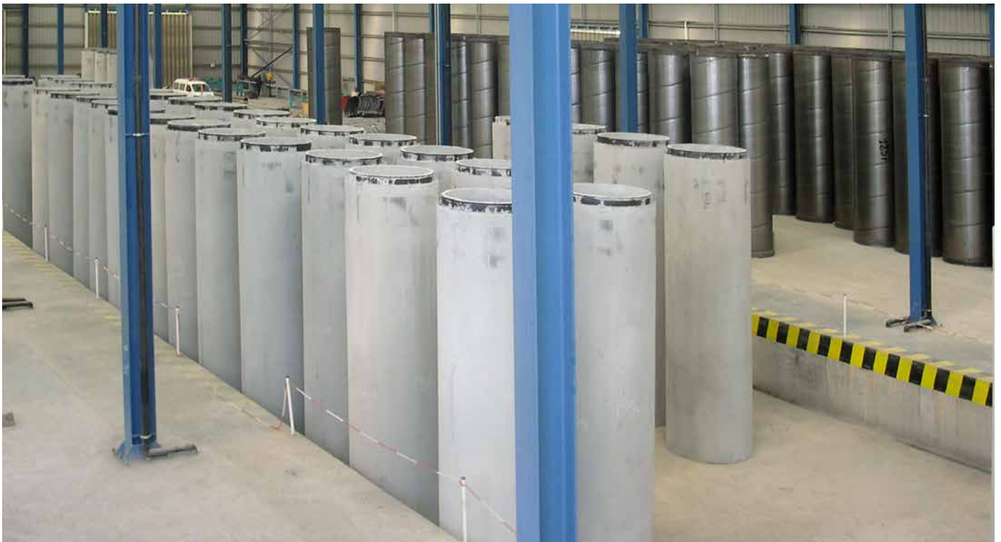
Finished Product and Steel Cylinder Storage Area
