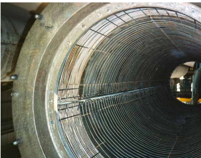
PCSP Mould reinforced by a cage and pre-stressed longitudinal wires
