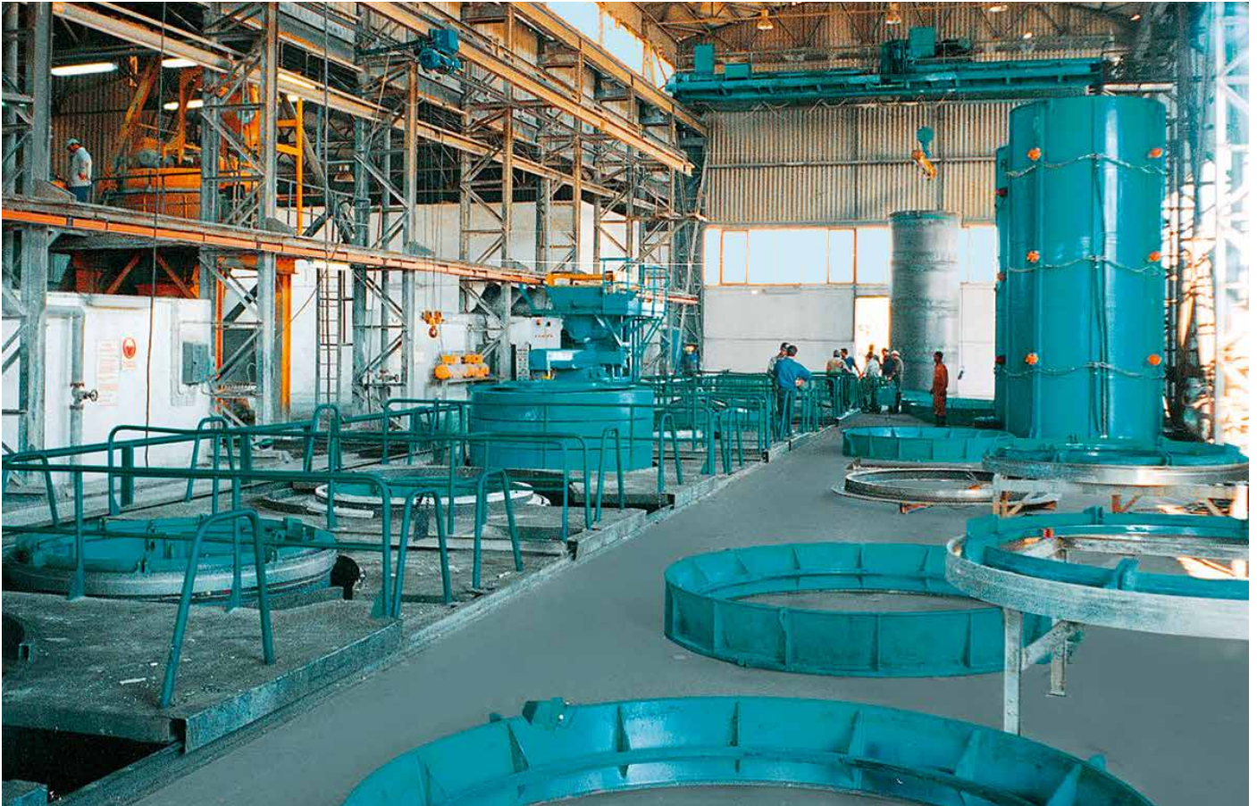
Mould Filling and Steam Curing Area
