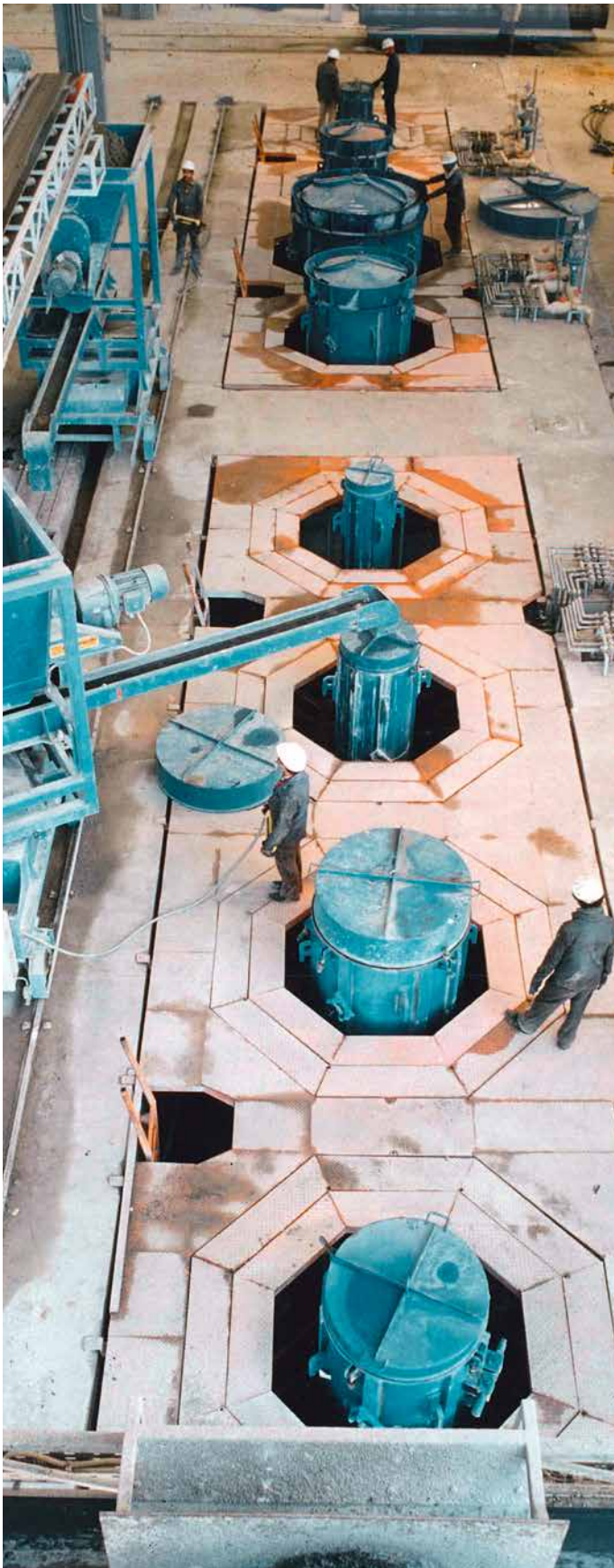
View on the PCCP Production Process Platform
